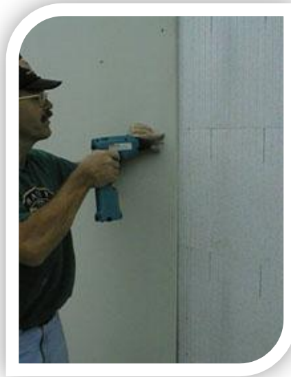
Example of fixing plasterboard Eco Block
