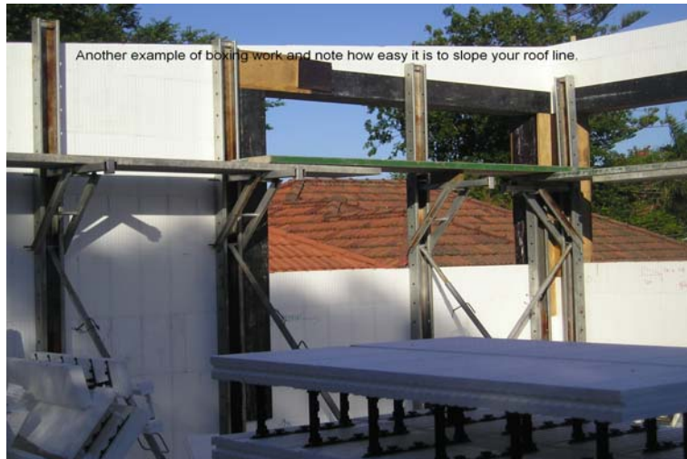
(9) Eco Block wall bracing system
