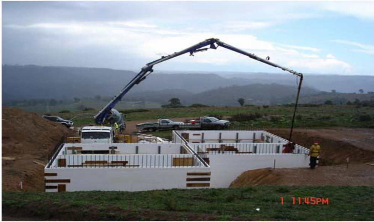
(12)Eco Block used as a retaining wall and basement
