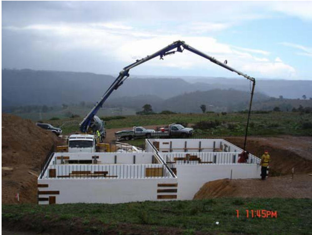
An example of Eco Block used as a retaining wall and basement
