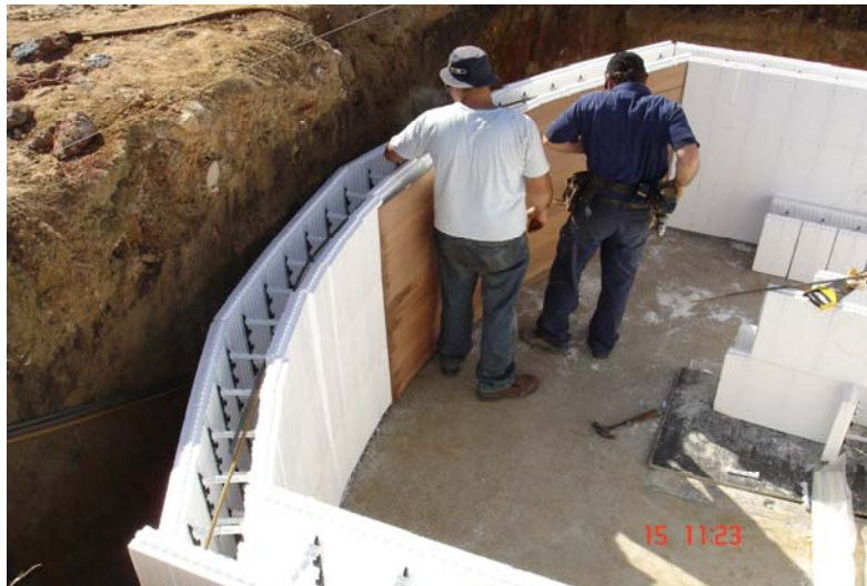
(11) Eco Block is used for a cellar, note how simple it is to curve and shape your wall.
