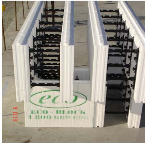
(2) Example of a 152mm thick concrete cavity
