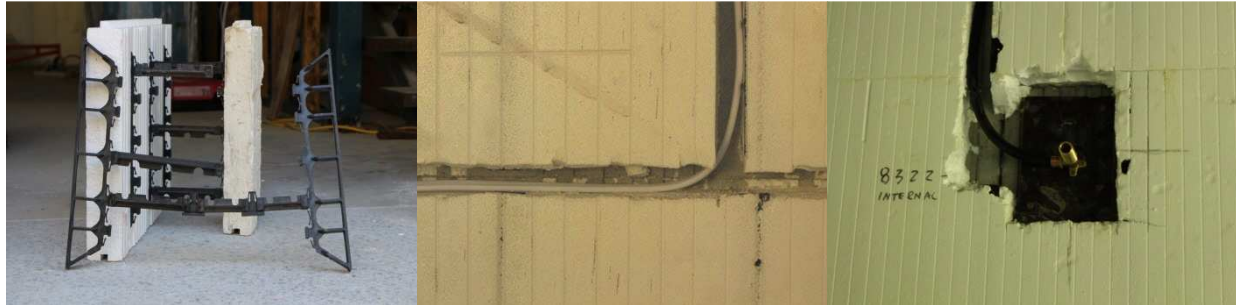
ICF Block with removed ribs and panel connectors
