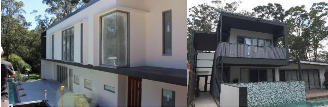
As an earlier experiment, the owner built a guest house on the block of land as the first stage in his building program. Part of the guest house was built with concrete walls and the other part with a conventional frame, both parts were built to a six star energy rating. To the owners astonishment walking from one section to the other revealed a profoundly higher level of comfort in the concrete section in both summer and winter.
