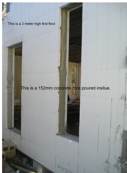
Formwork stripped away the following day
