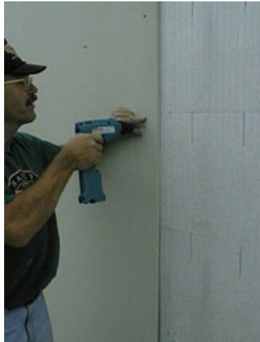
Example of fixing plasterboard Eco Block
