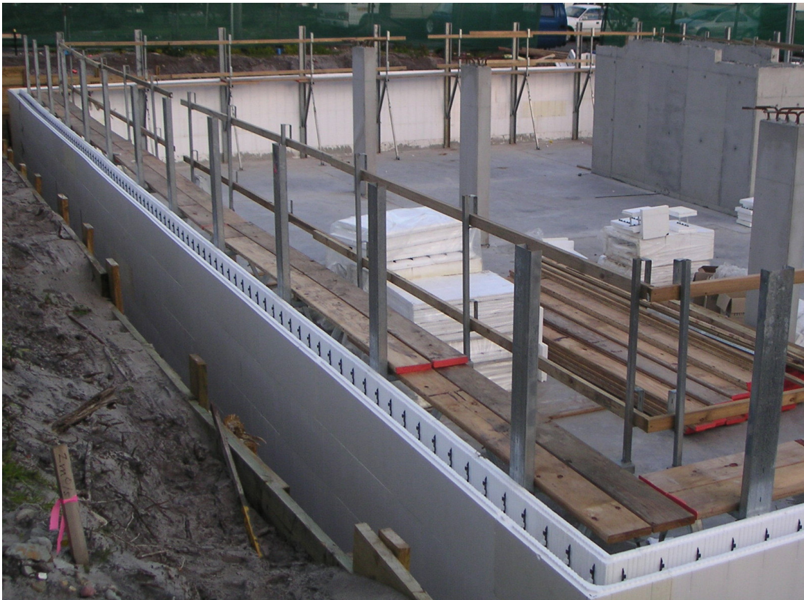
Eco Block Basement with braces erected, hand rails
