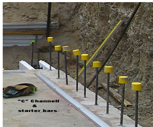
Photo "C" Channel placement
