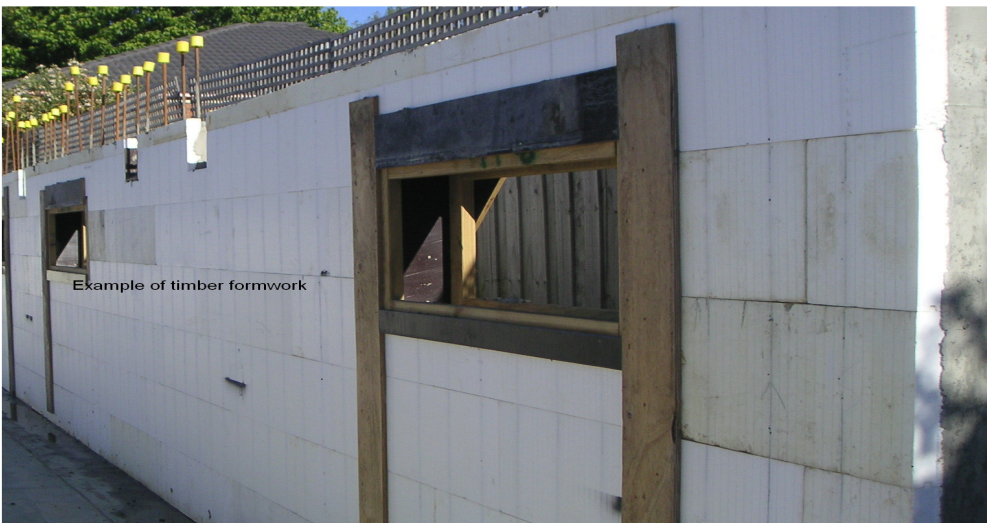
(Photo of timber formwork)
