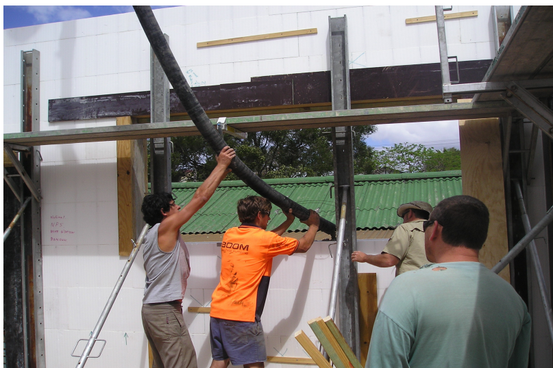
A typical crew of three with boom pump operator
