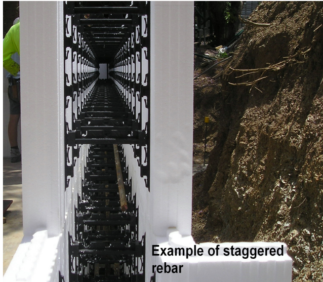
Photo: Example of Rebar Placement
